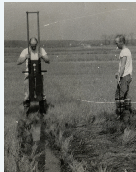
Fig. 2. The Botsford spade was patented to dig ditches more efficiently than with hand shovels.
