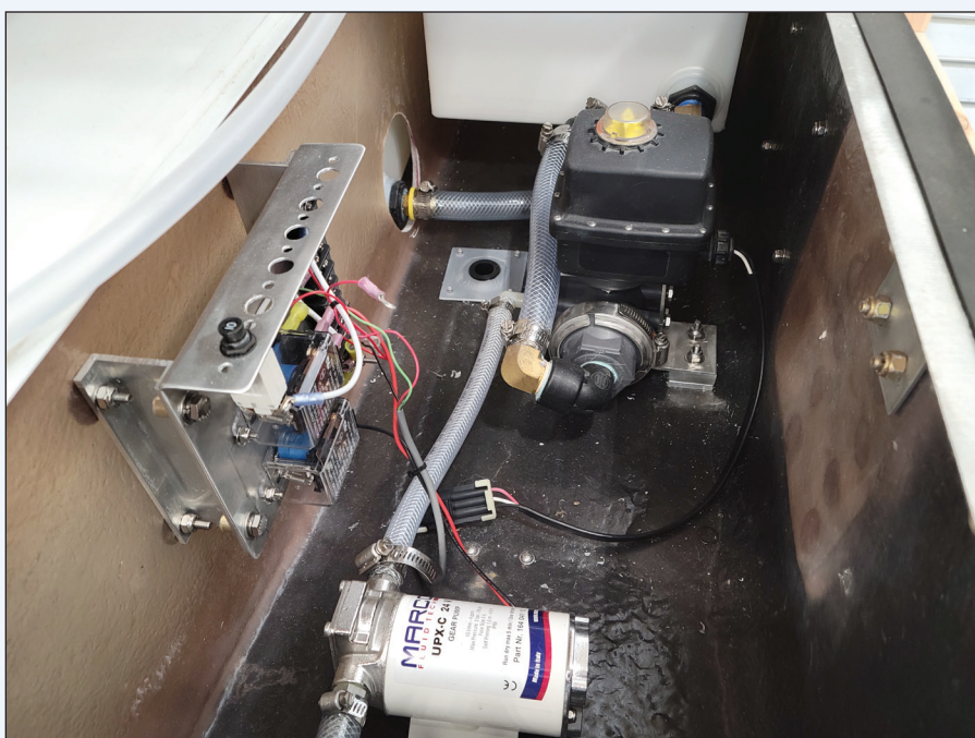
Fig. 1. The pump and valve setup currently used in MCMCD's chemical tanks.
