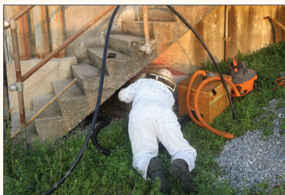
Fig. 4. Beekeeper removing honey bees from a city pump station in New Orleans.
