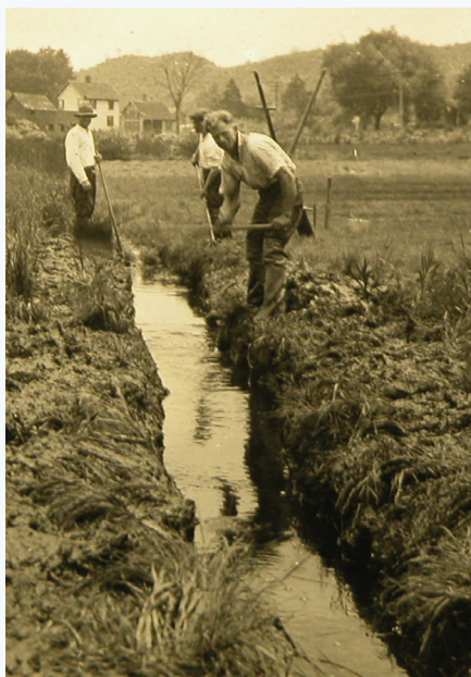
Fig. 3. CCC workers maintaining ditches.
